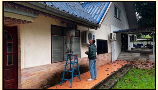
The children's room air conditioner was repaired.
